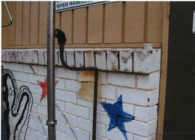
Figure 3: This brick wall is loose and unstable. (entry to pump house)
