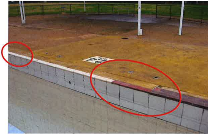
Figure 2: The circled areas of the Olympic pool deep end are both loose.
